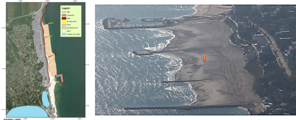
Figure 5. a.b. Eforie North before and after coastal protection works (2015/ 2016)
